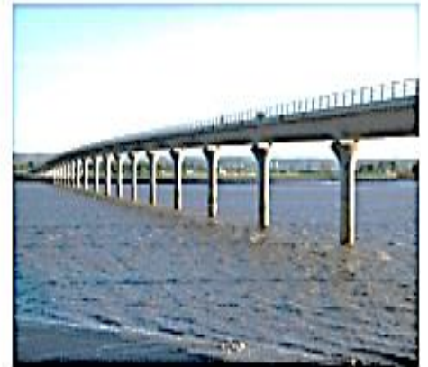
A bridge supported by columns
