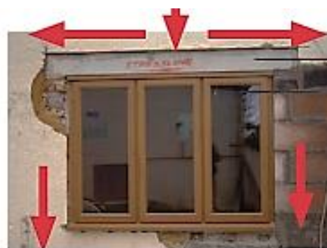
Figure 6 A concrete lintel used in the construction of a window
