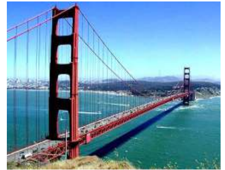
Golden Gate bridge - San Francisco
