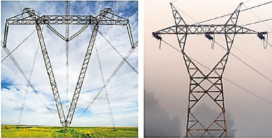
Figure 20 Electrical pylons are frame structures and come in a variety of designs.
