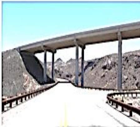
A bridge across a single carriageway
