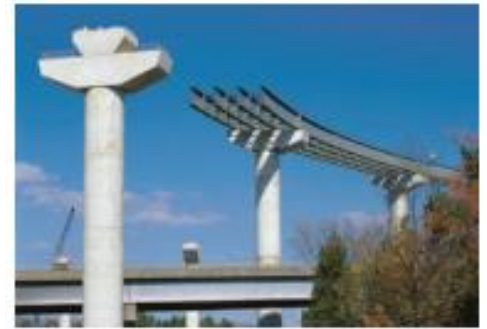
Figure 5 Steel I-beams being used in the construction of a highway.
