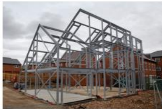
Steel roof trusses installed in a house
