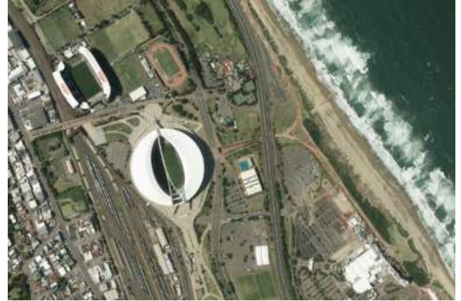
Figure 2.1 Showing a vertical aerial photo
