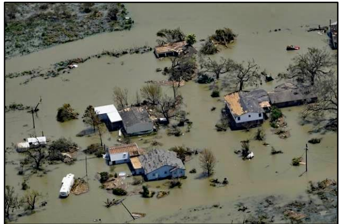
Storm surge damage in Cameron, Louisiana after Hurricane Laura on 27 August 2020
