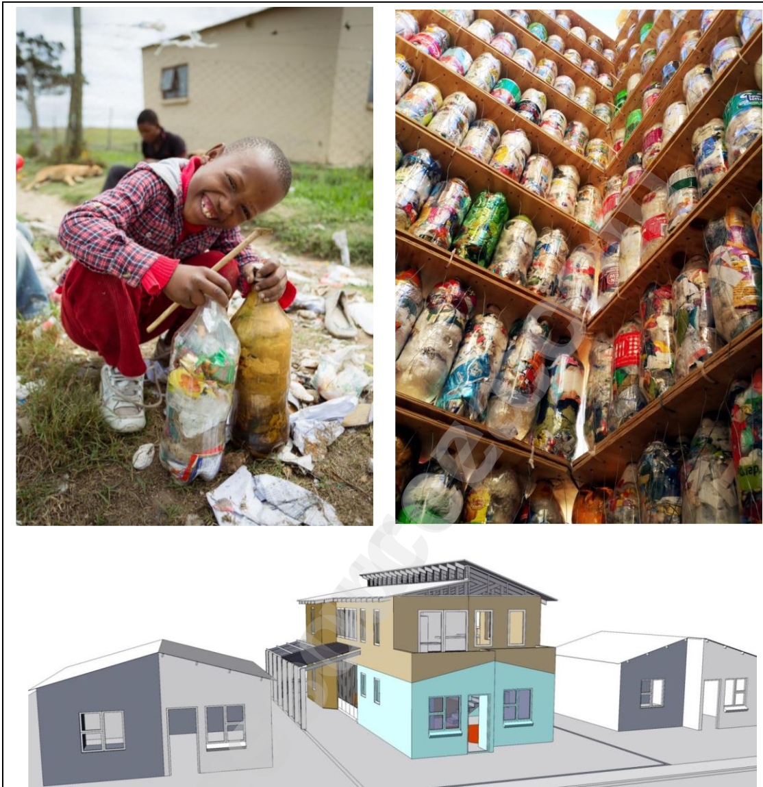
FIGURE A: Proposed 'Penguins Preschool', Walmer Township, Port Elizabeth. Walls are constructed of ecobricks, plastered and painted
